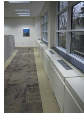
Fan coil units along the building facade
