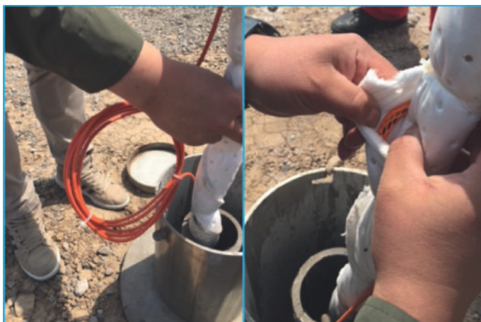
Figure 3: Example of installation with monitoring wells (main oil & gas operator in Asia)
