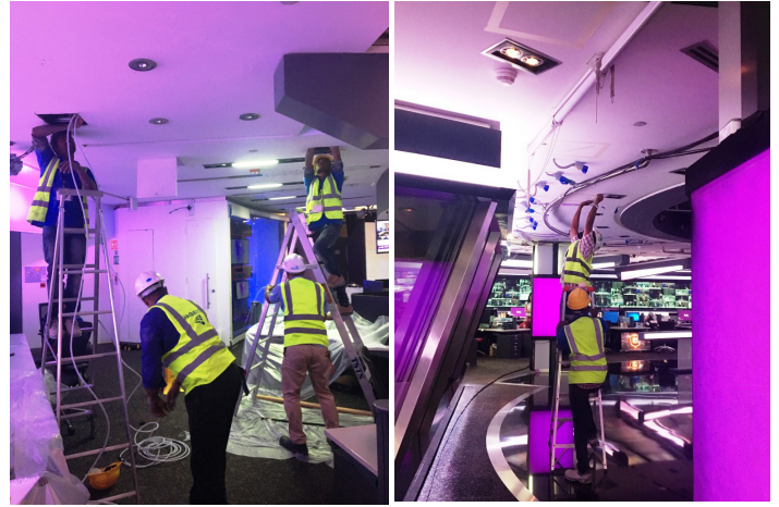
Installation of FG-ECB cables in the false ceiling of studio area
