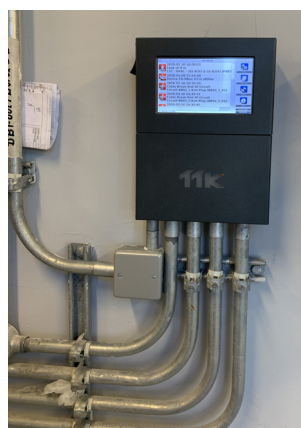
FG-NET Control Panel Installed On Site
