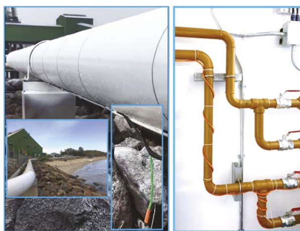
Figure 4. Examples of sense cable installation for aboveground pipes and transfer lines.
