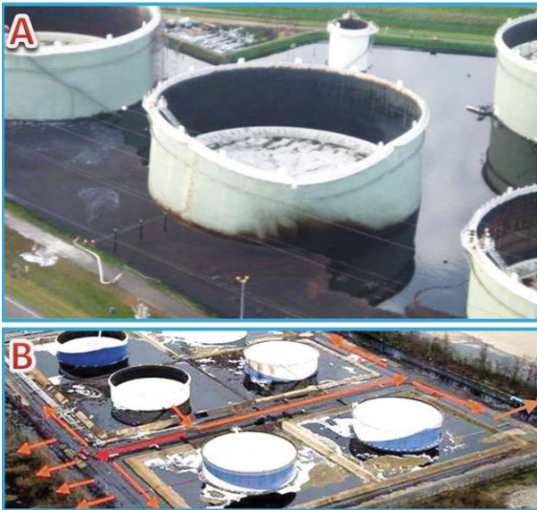
Figure 1. Rupture of crude oil storage tank in Kallo (a) and in Ambès (b).
