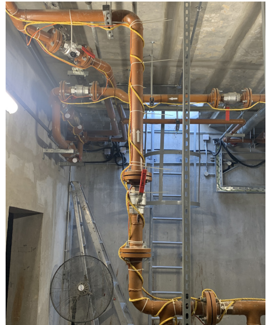
Installation of fuel sensing cables on a vertical fuel pipe
