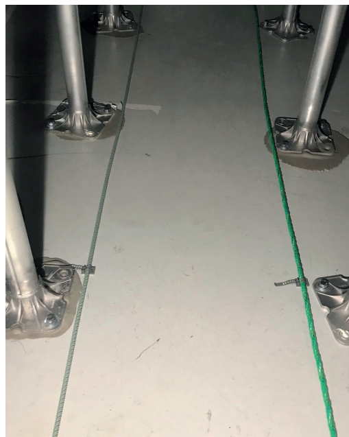
TTK fuel and acids sensing cables under the raised floor of the laboratory
