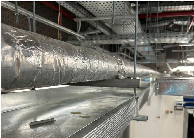
Overhanging chiller water pipes with drip tray
