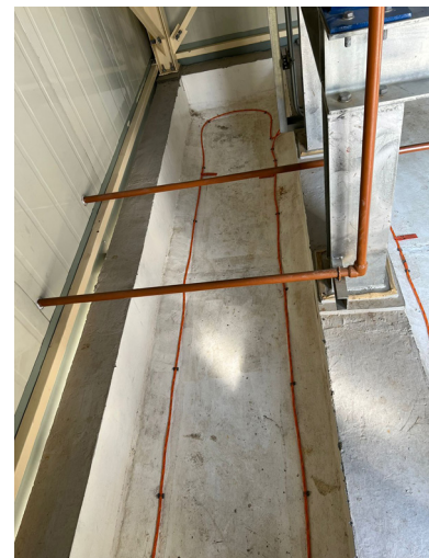
TTK oil fuel sensing cables (FG-OD) installed under a day tank
