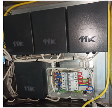
Four FG-BBOX Satellite Panels Installed On Site
