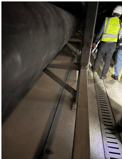
TTK Water Sensing Cable Installed Near Water Pipes
