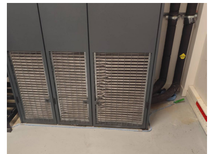
TTK water sense cable installed around critical equipment
