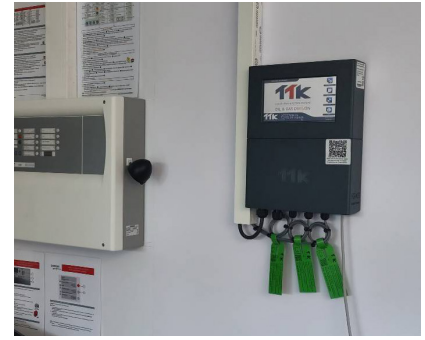
TTK FG-NET panel installed on site
