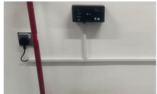
TTK custom-built FG-A kit panel installed on site
